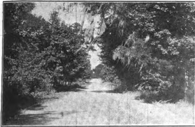
The new Waters road, ready for use
